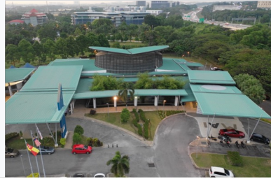
MARii Main Office Block 2280, Jalan Usahawan 2, Cyber 6, 63000 Cyberjaya
