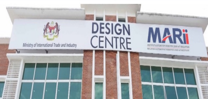
MARii Design Centre (MDC) Jalan Jasmine, Bandar Bukit Beruntung, 48300, Selangor (Relocation)
